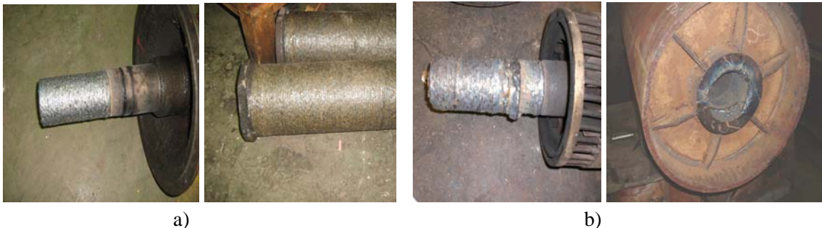
Figure 1. Visual control; a) Details repaired by welding successfully; b) Details that are not repaired by welding properly
