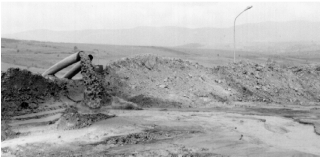
Figure 2. Details showing hydraulic ash disposal at the existing landfill nearby thermal power plant
