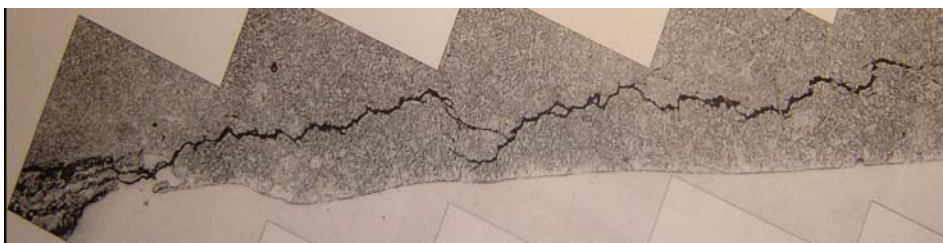
Figure 1. The cracks in the heat affected zone welded joint the tank connection
