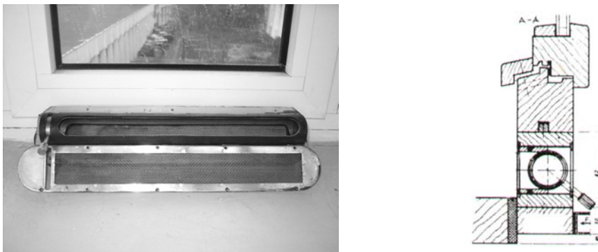
Figure 2. Airing device with concentric cylinders
