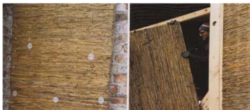
Figure 3. Isolation of the outer wall of reed [4]
