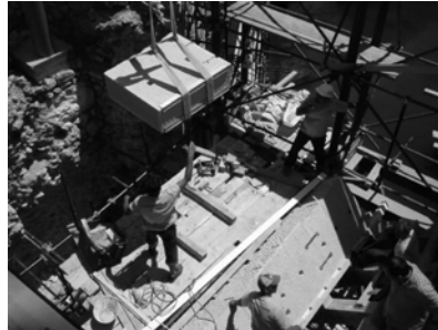
Figure 3. Assembling of the load bearing arch
