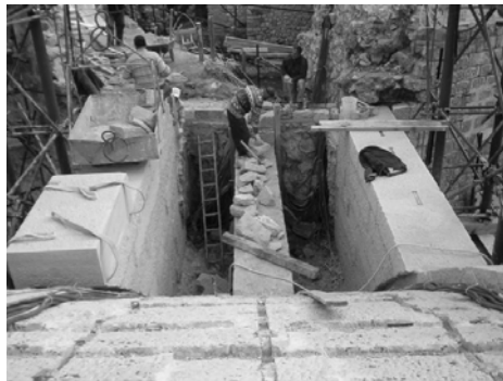
Figure 7. Assembling of the spandrel walls and middle rib
