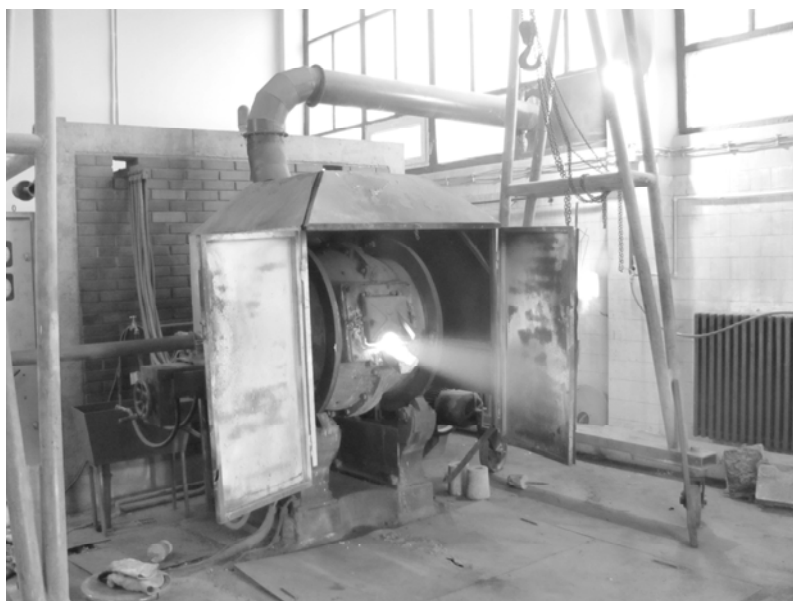
Figure 1. BIRLEC furnace for melting spent automobile catalyst
