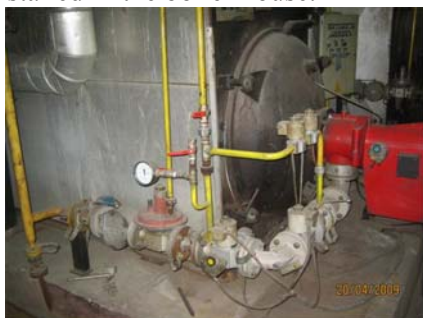
Figure 4. View on the old boiler
