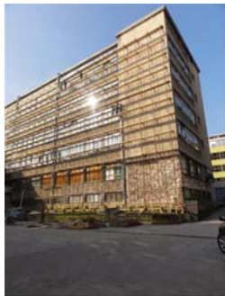
Figure 2. View on the west MEF building before
