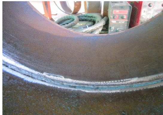
Figure 5. Inner surface of root pass (steel pipe)
