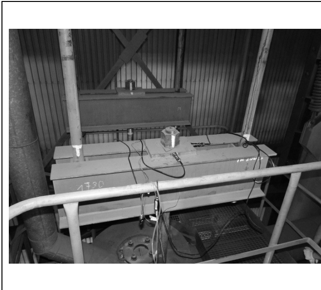
Fig. 4. Original separator mounting system.
