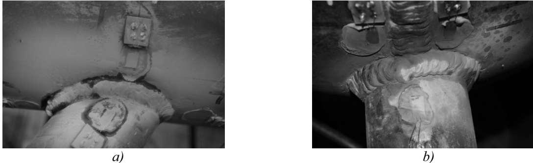
Figure 4. Crack position of the branch connection sample without reinforcement (a) and with split sleeve (b)
